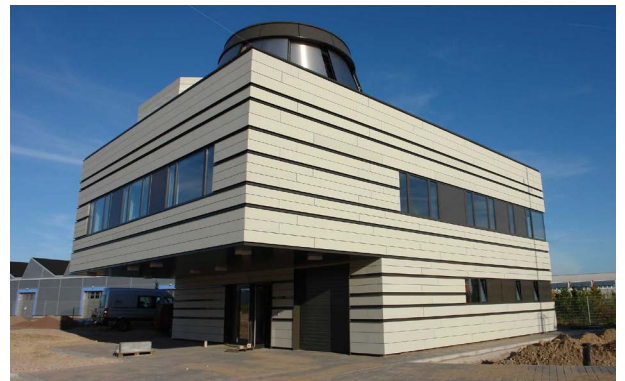
An KL-P-034 ventilates the new laboratory building of the Fraunhofer Institute in Ilmenau.
